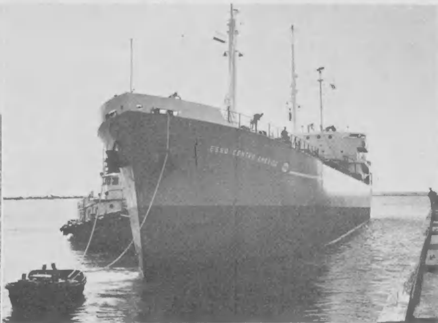
THE ESSO Venezuela left Aruba in November, 1961, after it was towed here by the Esso San Nicholas. Repairs to the weathered, unkempt vessel enabled the T-1 to travel to Hamburg, Germany, where it was refurbished to a bright, efficient ammonia carrier, and renamed Centro America. ESSO VENEZUELA a laga Aruba na November 1961 despues cu el a worde getouw door di Esso San Nicolas. Reparacion na e barco cu tabata afectá pa condicionnan di tempo a permiti e tankero T-1 pa viaha pa Hamburg, Alemania, na unda el a worde renobá pa un bapor.
